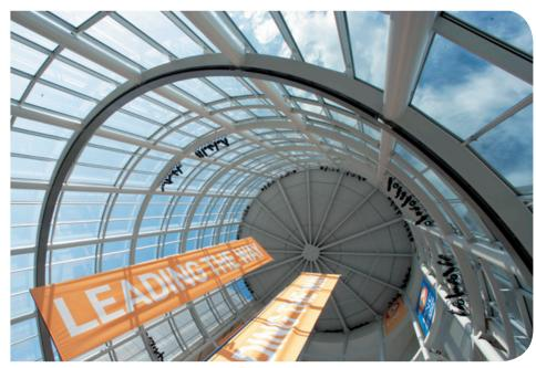
Solarban® 60 glass by Vitro Architectural Glass transmits light into Prudential Center through two 110-foot-tall glass and steel cylinders.
