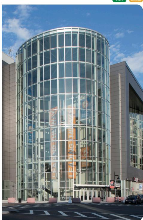
The Prudential Center in Newark features vast expanses of clear *Solarban*® 60 glass by Vitro Architectural Glass (formerly PPG glass), which connects the building to the local streetscape and helps control its lighting and cooling costs.
